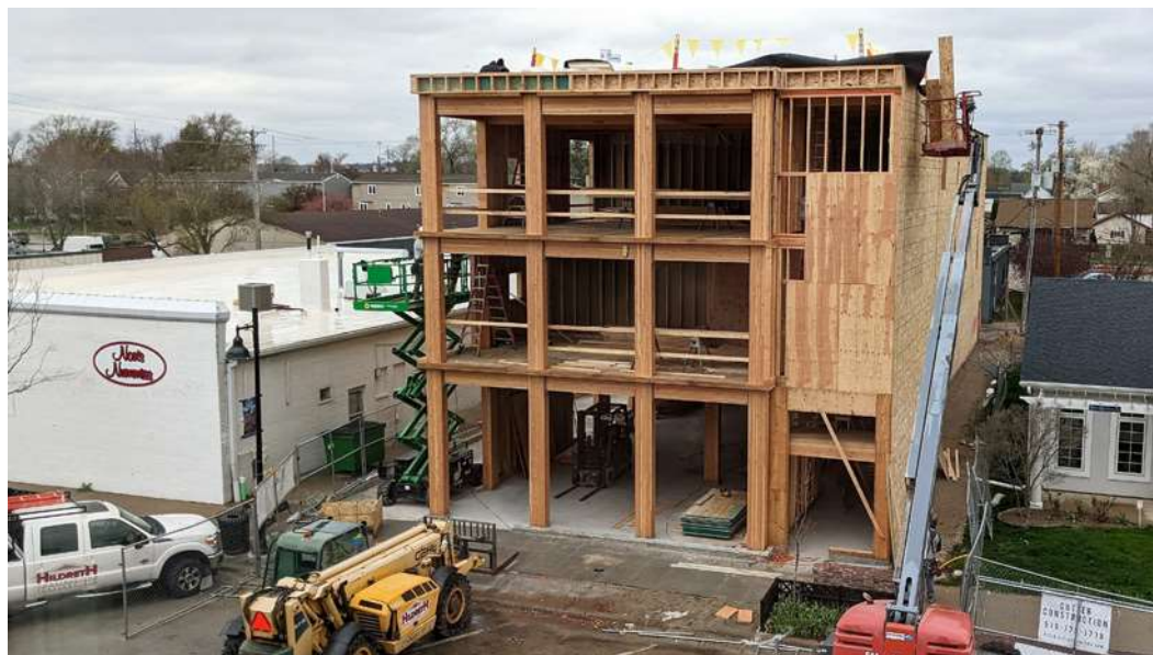
West Valley Junction New Construction
