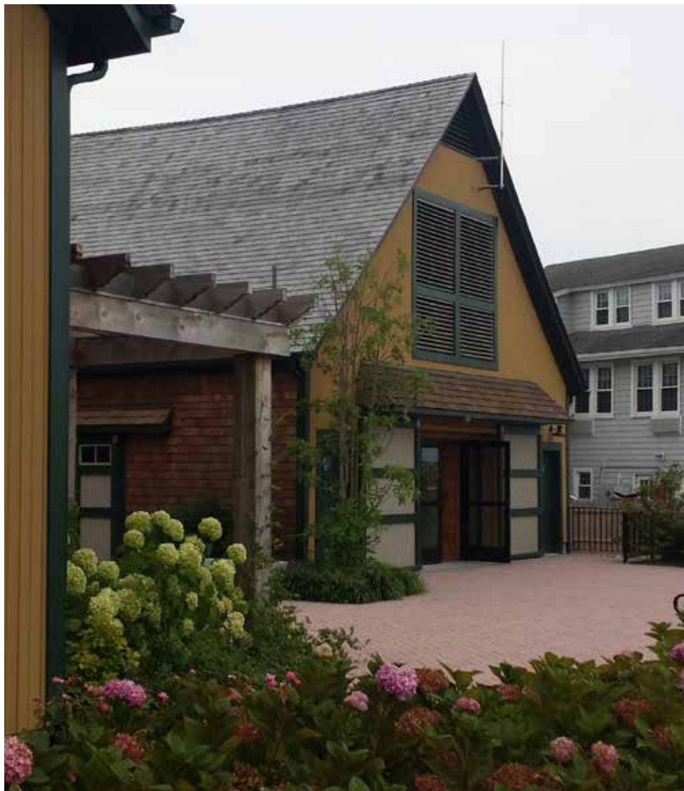
Figure 6: The mechanical room was relocated to the upper floor at the back of the building, discernible in this photo by the louvered vents. Photo: Jennifer Wellock/NPS
