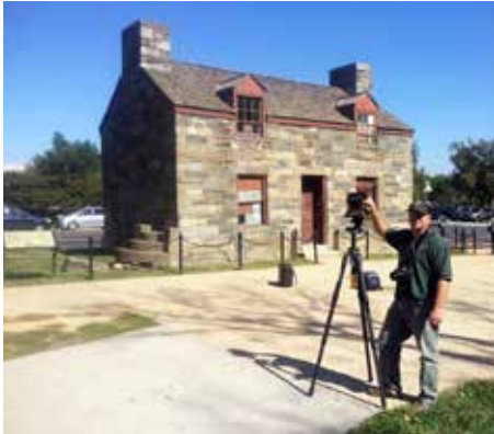
[15] Surveying and documenting existing building conditions is always recommended prior to implementing an adaptation strategy. NPS Historic American Building Survey (HABS) staff photograph the 1833 Lockkeepers House on the National Mall in Washington, DC, prior to the building's relocation and restoration. Photo: Heritage Documentation Programs/NPS
