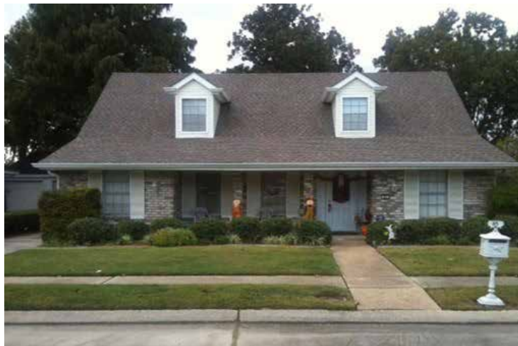
(a) Photo: Rubion Construction Co., LLC
