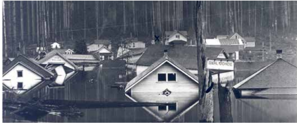
[2] Communities have historically employed numerous methods in response to flooding, including wholesale property buyouts and removal. The 1915 flood in Cedar Falls, WA, led to an early example of a “buyout zone” to remove buildings damaged and at risk. Photo: Snoqualmie Valley Museum Collection: PO.074.0786
