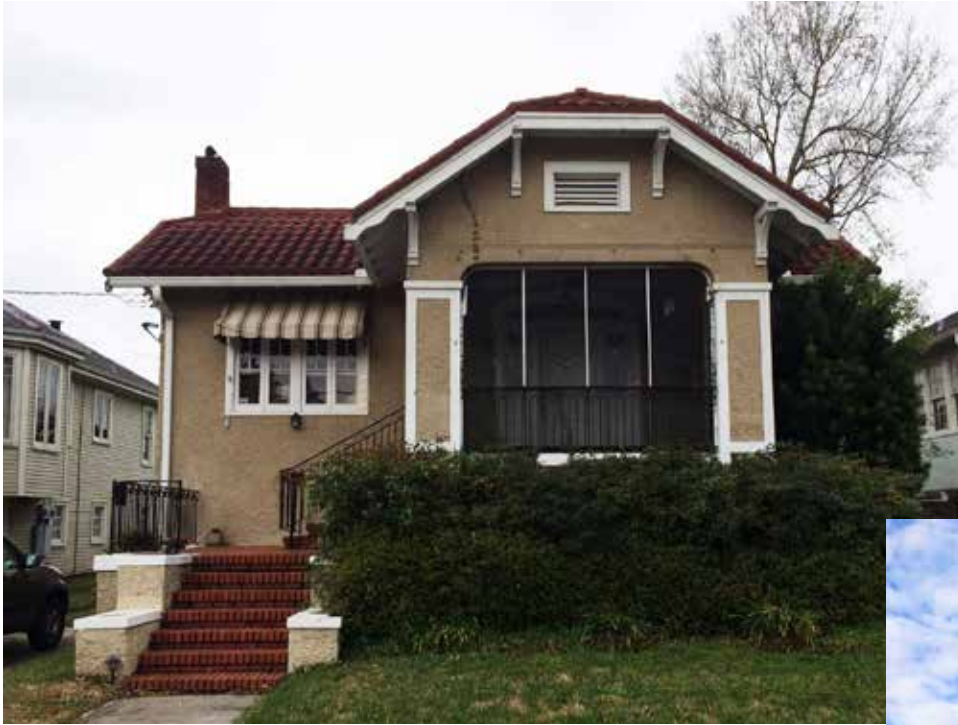
(a) Photo: Rubion Construction Co., LLC
