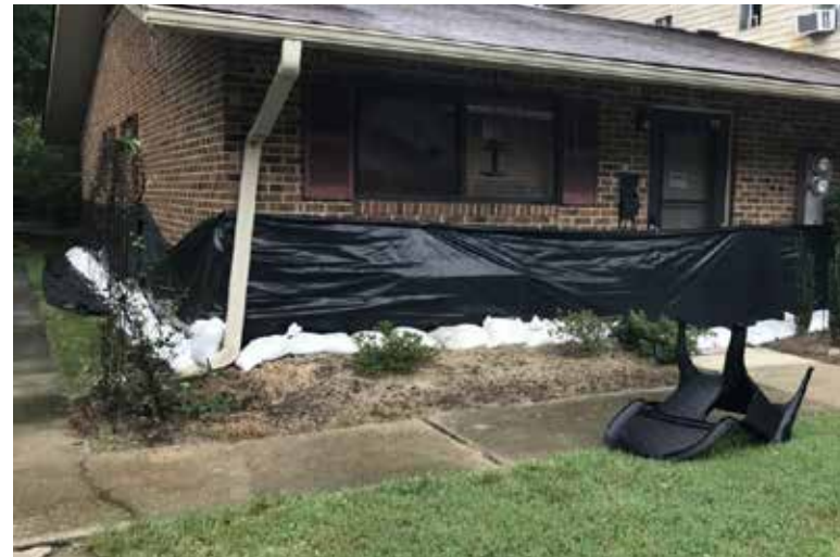
[23] A combination of different temporary measures can be an effective short-term solution to flooding. In this case, a building wrap of waterproof fabric is anchored by sandbags. Photo: Chapelboro.com
