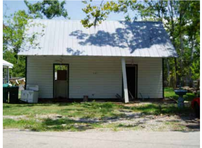
(a) Photo: Rubion Construction Co., LLC
