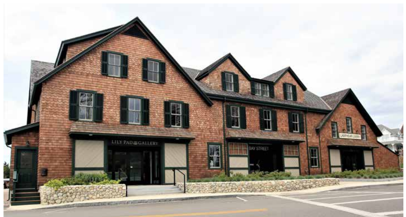
Figure 5: View of the building after the floodproofing and rehabilitation project was complete. The historic barn doors and many historic windows were preserved. Damaged or missing shingle siding was replaced in kind. The foundation is now two feet taller than it was at the start of the project. Wet floodproofing of the first floor provides additional resiliency and protection for floods that exceed the new elevation height. Photo: Pariseault Builders
