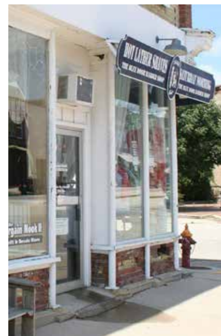
Figure 3: The historic storefronts and brick bulkhead were extant before floodproofing work began on the Driver Opera House. Photo: KONTEXT architects llc
