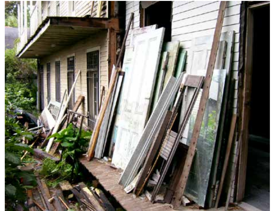
[120] If a property is demolished, carefully salvaging historic materials can help other historic properties undergoing rehabilitation and give a 'second life' to these otherwise lost materials. Photo: Jenifer Eggleston/NPS
